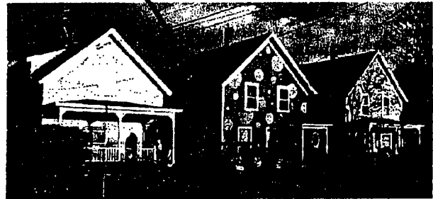
274, 276 and 278 Colchester Avenue Note existing aerial lines between 274 and 276
